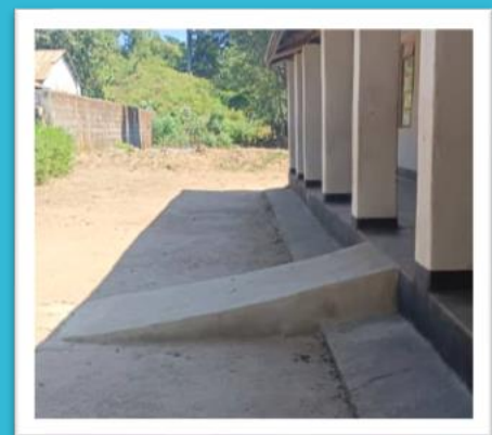
A newly constructed ramp at Lubwe school following SBC activities.
